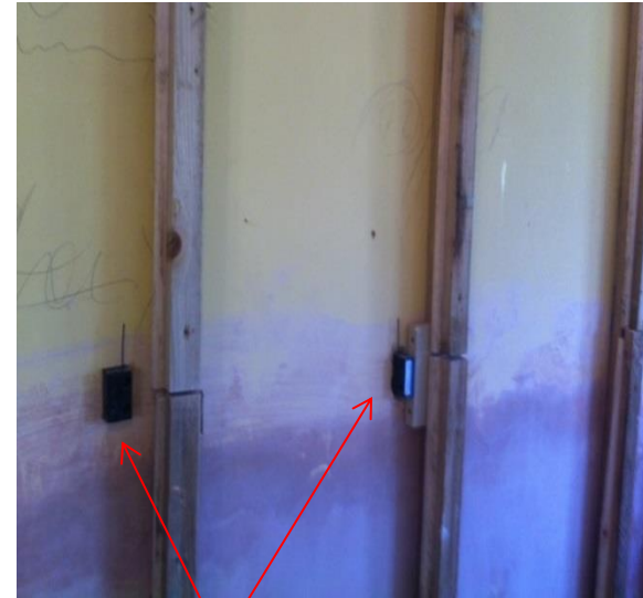
Moisture sensors (in the timber studs)
