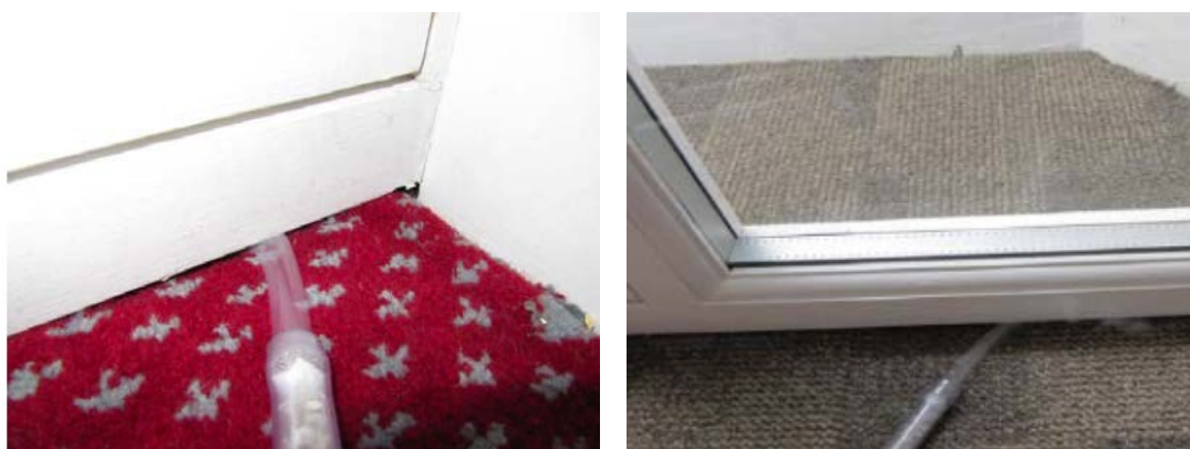
Figure 3 Secondary glazing frame. Air is drawn through the gap between the secondary glazing and the carpet.
