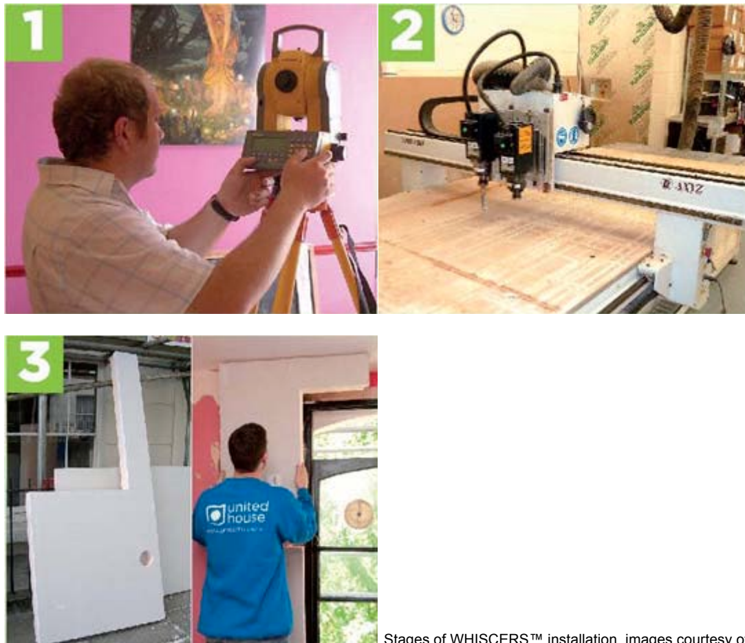
Stages of WHISCERS™ installation, images courtesy of United
