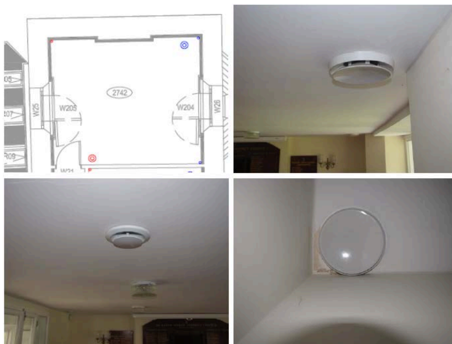
Figure 44 i) top left-excerpt from Passivent drawing. ii) top right-a supply air valve used as extract.
