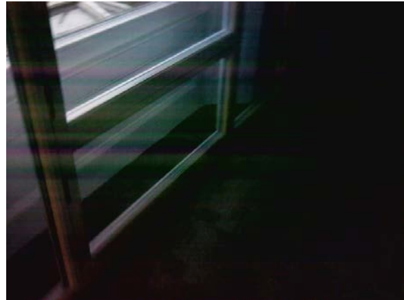
Figure 35 Room F21. The image shows heat loss through the edge of secondary glazing. The smoke test also shows the smoke drawn under the secondary glazing.
