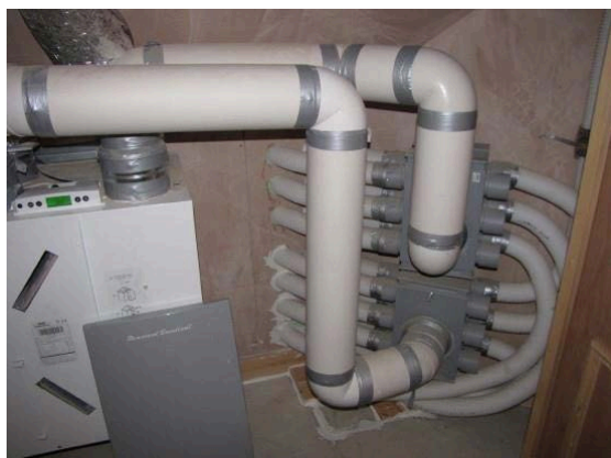
Figure 45 Supply and extract ducts (rigid) serving the supply (top) and extract (bottom) plenum manifolds
