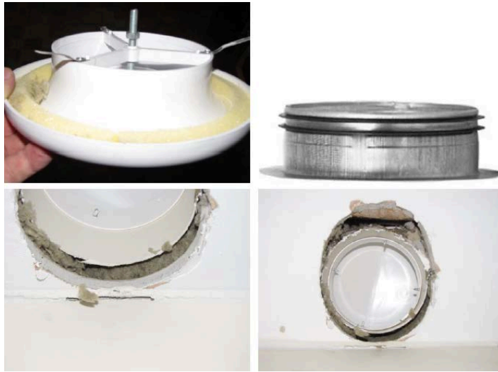
Figure 43 i) top left-diffuser showing untightened locking nut. ii) top right-an example of a gasketed flange spigot. iii) bottom left-gap between duct end and ceiling. iv) bottom right-oversized cut outs in plasterboard.
