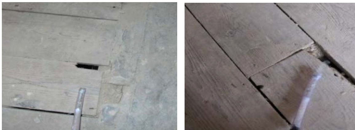
Figure 7 Gaps in floor. Smoke drawn under floor.
